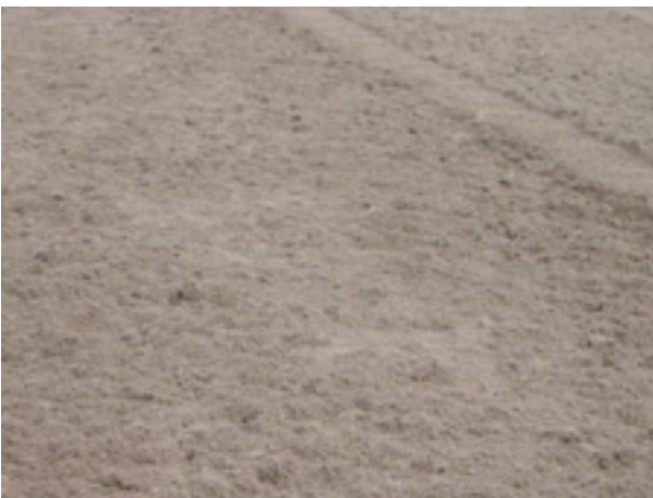
Levelling reinforced Loksand
