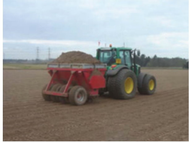
Laying fibre reinforced sand
