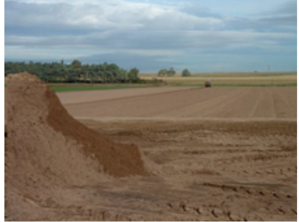
Laying of reinforced fibresand
