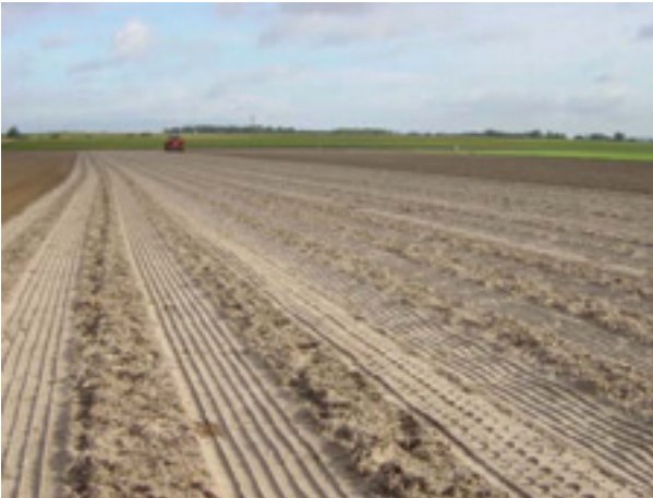
Laying reinforced Loksand
