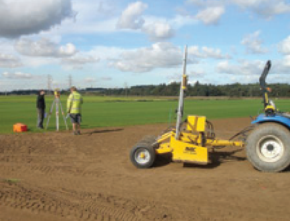
Laser levelling of surface
